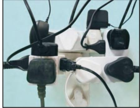
Fig. 11.14: An overloaded power socket
