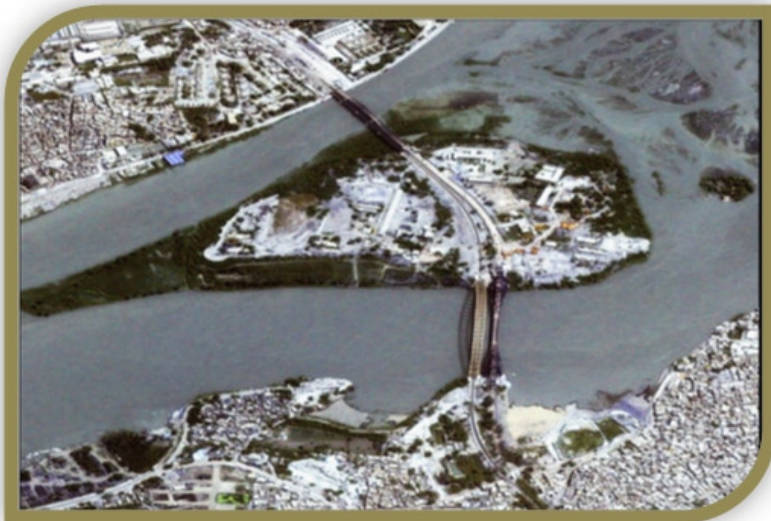
Figure 12.12: Ayub Railway Bridge over Indus River at Sukkur (As seen from space - Satellite View)
