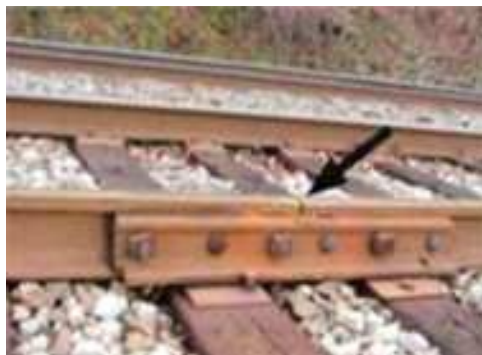
Fig. 9.19 A rail expansion joint, indicated by arrow
