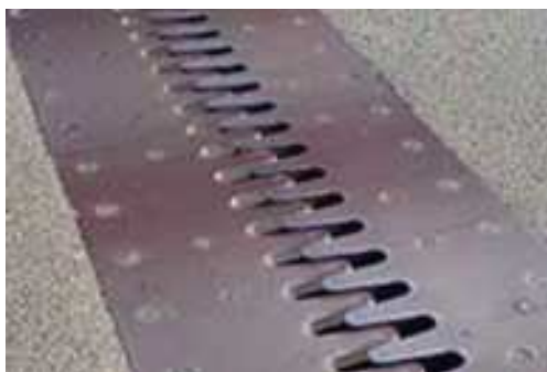
Fig. 9.20 A bridge expansion joint
